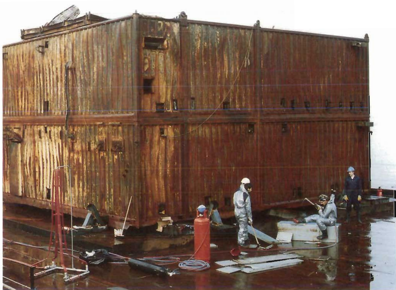
Plate 23 Accommodation modules at Flotta after recovery from the seabed — 2: the Additional Accommodation West (AAW).
