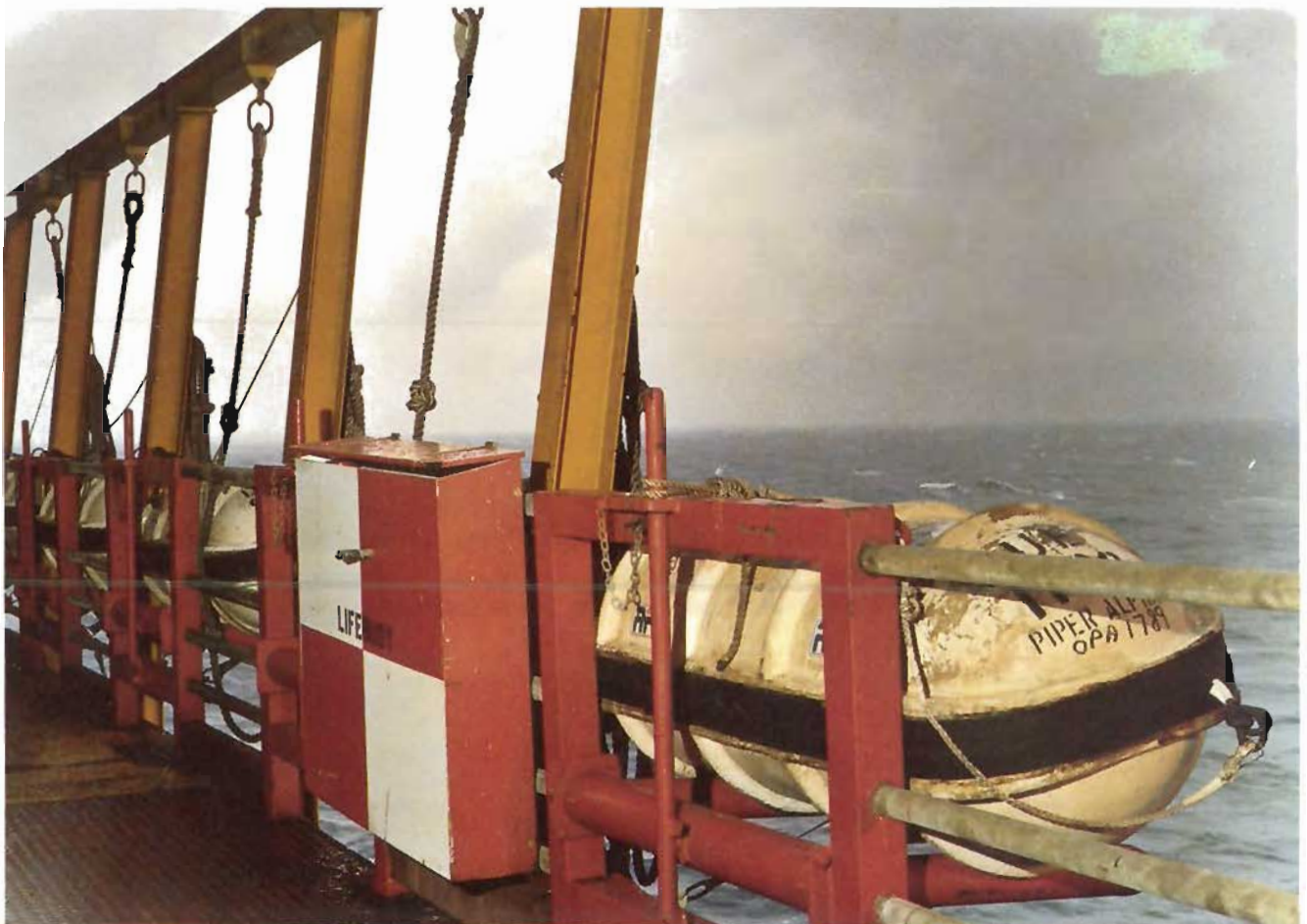
Plate 12(b) A Piper liferaft on its launching platform.
